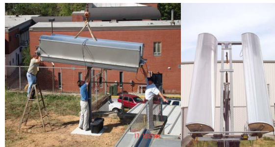
Figure 6: Entech Solar SunLine during installation at Auburn University.
